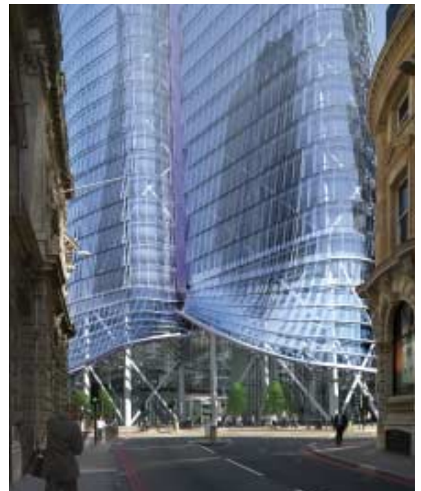
3. Complex canopy entrance to the Bishopgate Tower.
